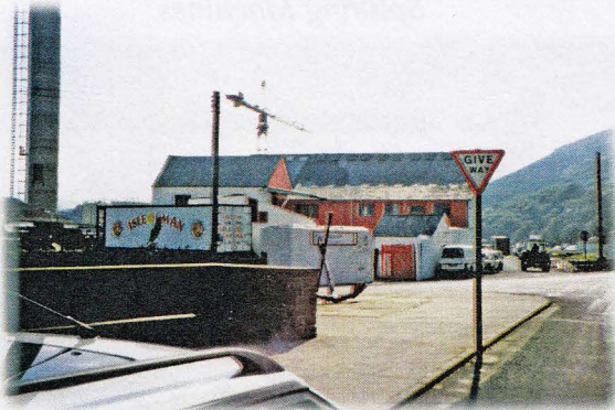
Mill Road Premises September 1993
