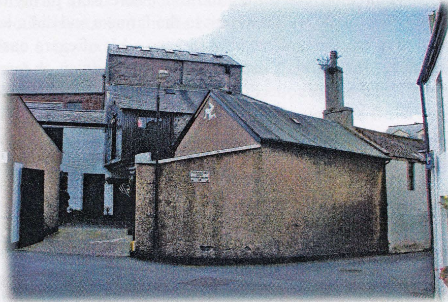
Michael Street Yard
